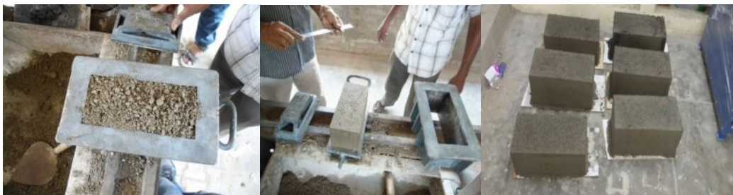
(a) Paver Block Mould (b) Casting of Paver Block (C) Curing of GPC blocks
